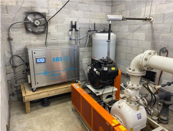
The EBS-Di unit utilizes a customized proprietary active state soil microbiology, custom-tailored by EBT to Silver Spring’s wastewater, that is autonomously delivered into their collection system using a patent-pending process which generates and activates the microbiology consortium. The microbes perform without oxygen, are highly adaptable and immediately went to work, rapidly dominating Silver Spring’s system.
